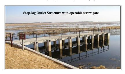
**PROJECT COMPONENTS:** Approximately 9 miles of earthen embankment, an outlet control structure, rock lined emergency spillway, and an enlargement of a portion of Ditch 200.
