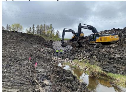
Excavating the outlet channel and installing riprap (Looking South)
