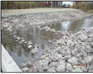
Riprap riffles downstream of concrete structure
