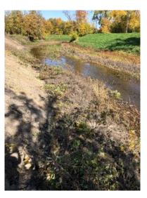
These photos are areas along State Ditch #83 that were part of the Toe Wood Sod Mat Installation It was installed to protect the integrity of the ditch bank and stop or slow down bank sloughing and erosion.
