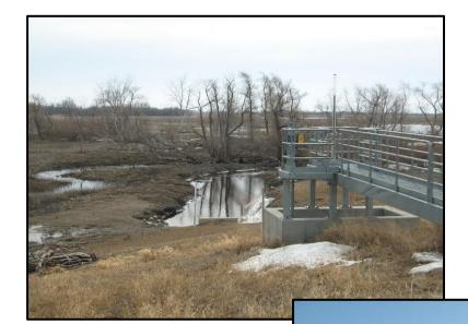
Example of a "Dry" Impoundment. Stored flood water is released as soon as downstream channel conditions are acceptable to pass flows.
